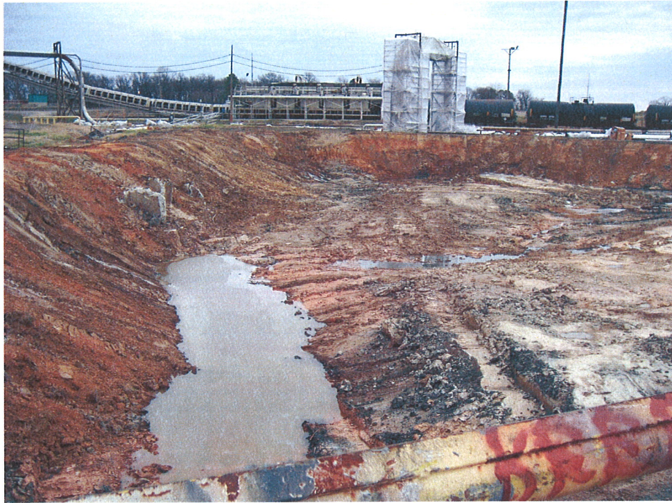
Photo 1. Excavated pond January 8, 2014.
